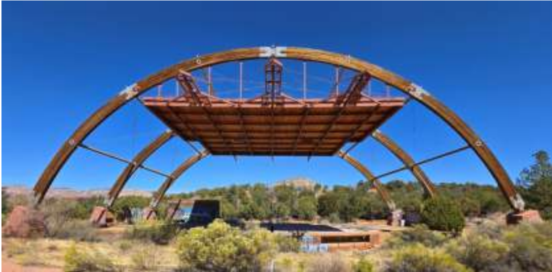
Figure 1A: View of structure from the south
