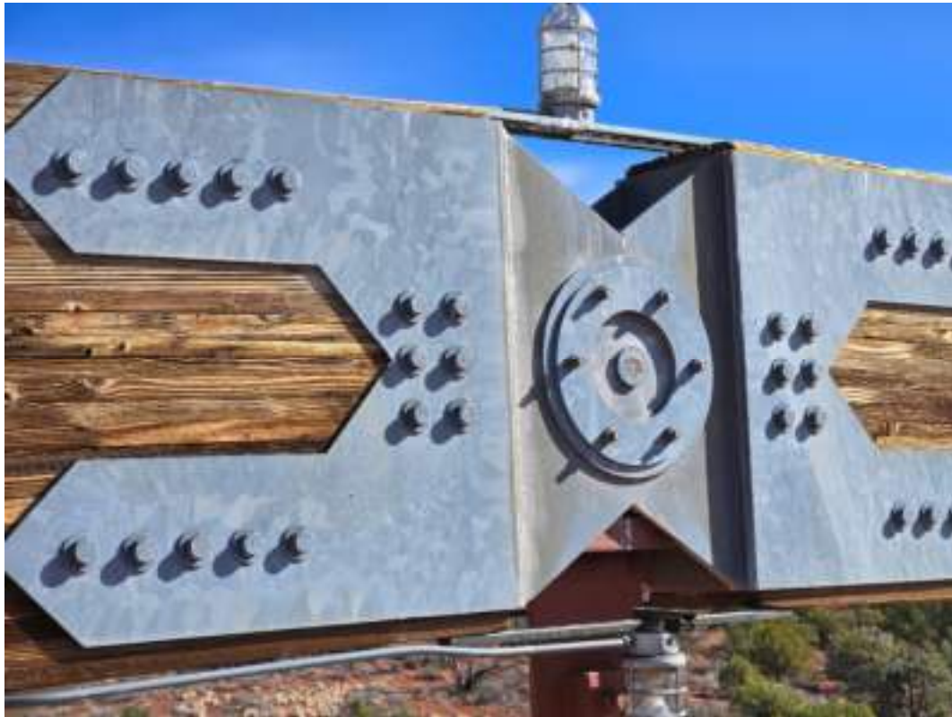
Figure 2F: View of bolted hinged connection
