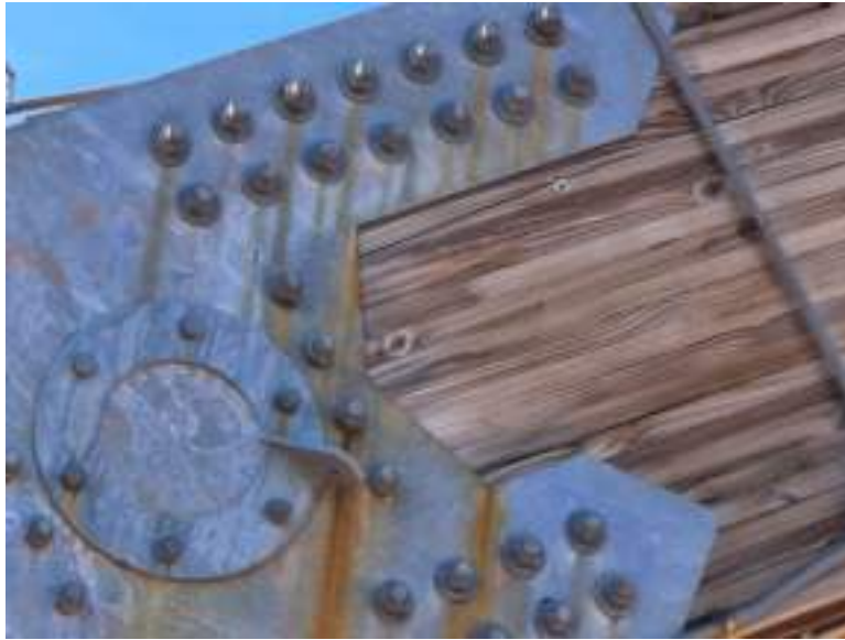
Figure 2E: View of bolted splice connection
