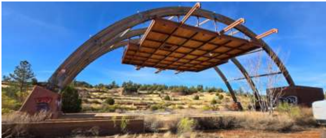
Figure 1B: View of structure from the north
