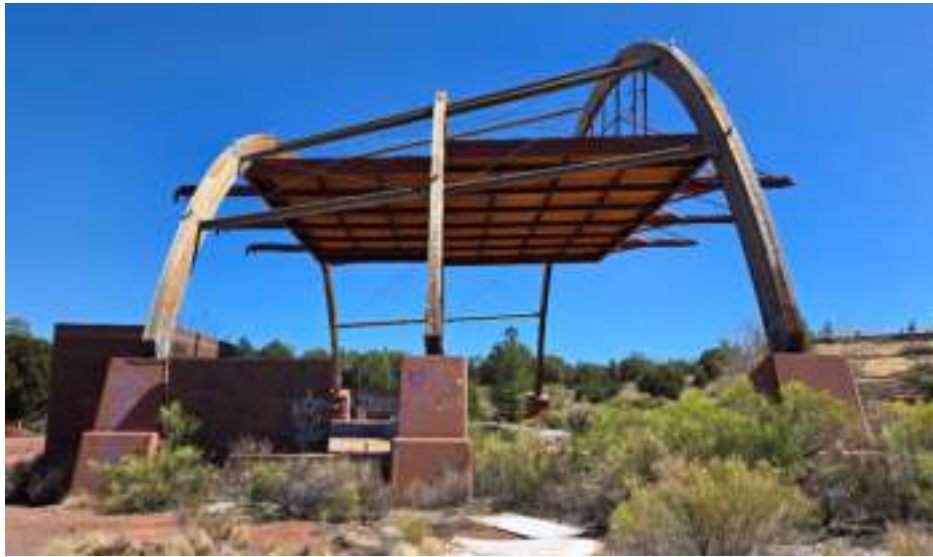
Figure 1C: View of structure from the west
