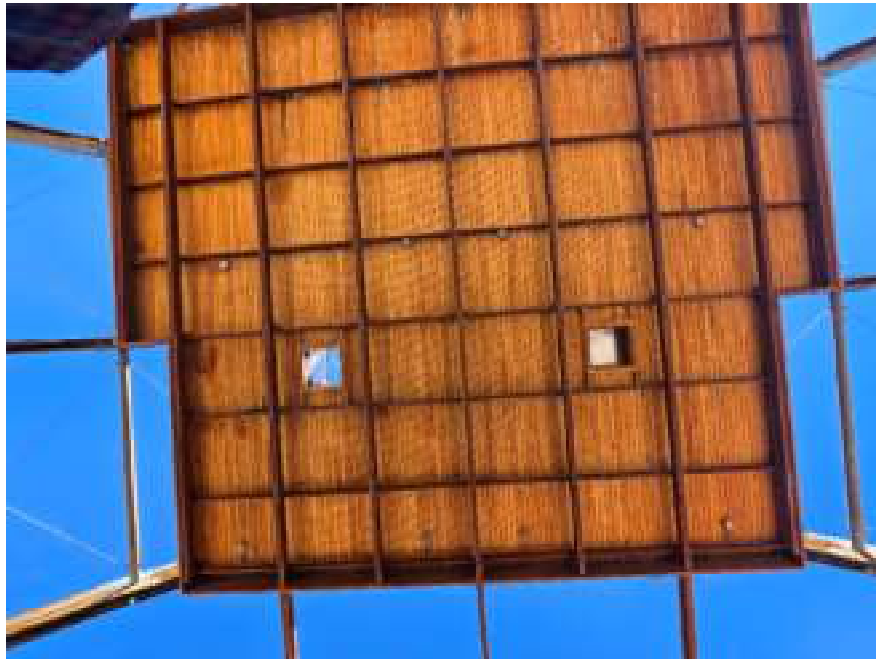
Figure 1D: View of underside of canopy
