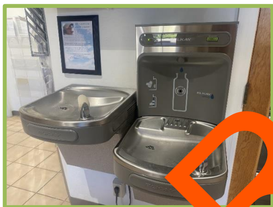
Action Item 4.3.1 Water bottle filling station to reduce plastic water bottle at city facilities
